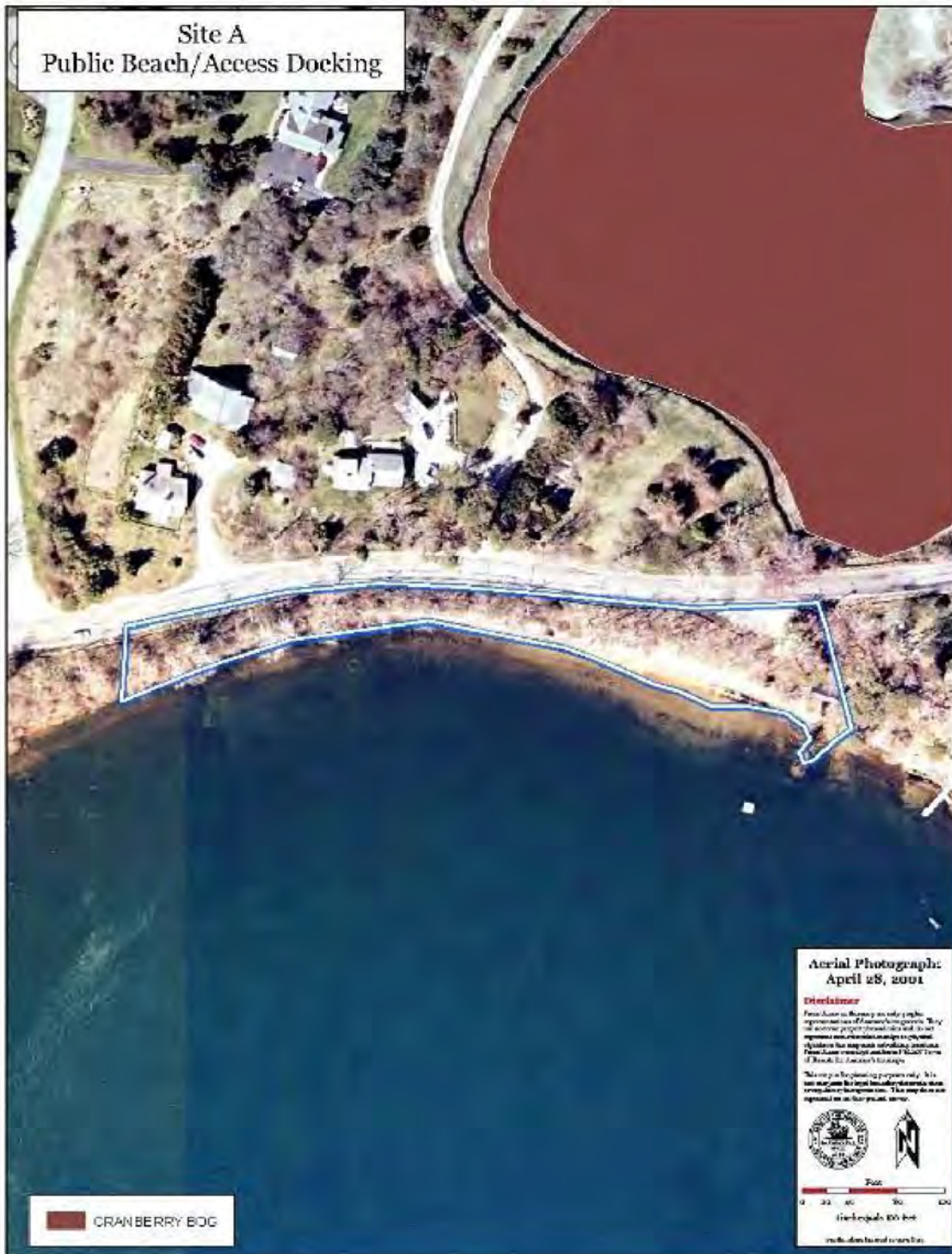
Figure 5. Access Point A, Potential Chemical Storage and Barge Filling Area
