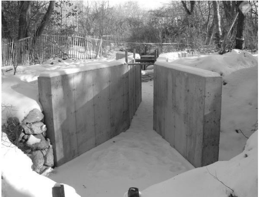
View through the new reinforced-concrete ladder of the Middle Pond Herring Run looking upstream towards the channel leading to Middle Pond. Photo by Emory Anderson
