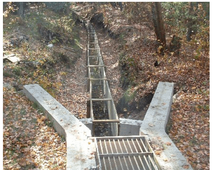
View downstream from Middle Pond herring run ladder showing 140 ft of newly installed pressure-treated lumber side walls.
